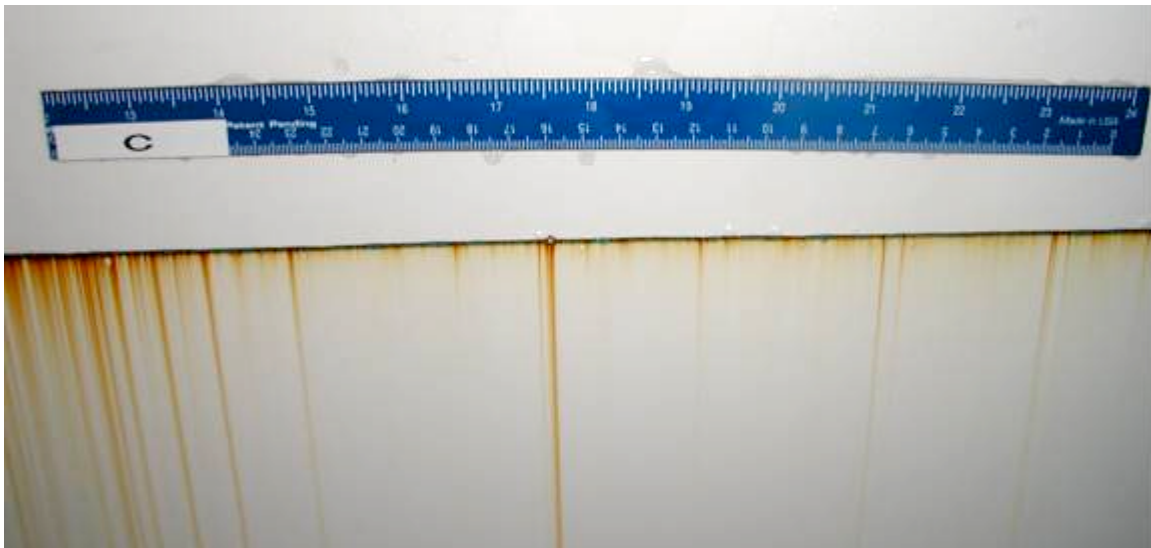
Figure 8. Control panel appearance (Experiment One)
